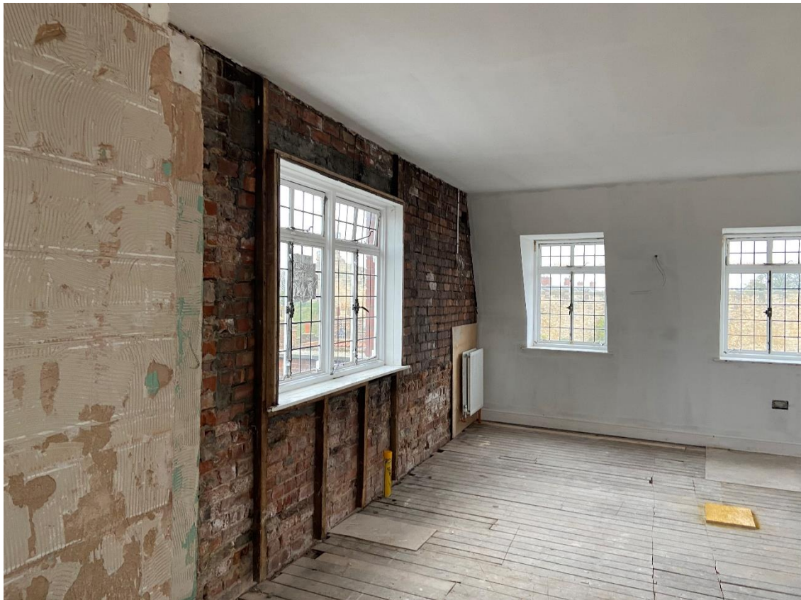
Window to be altered to form door with internal steps adjacent
